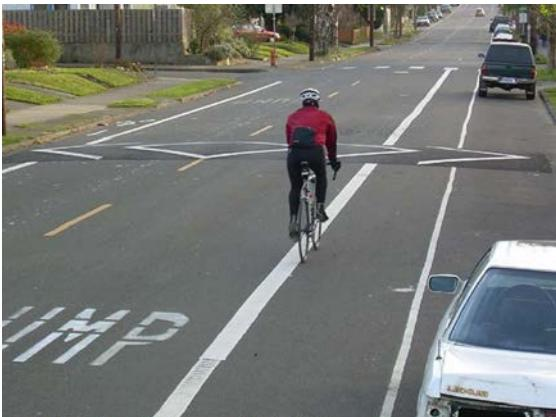
Figure 3.10.1. Speed Hump with Bicycle Lane and On-Street Parking
